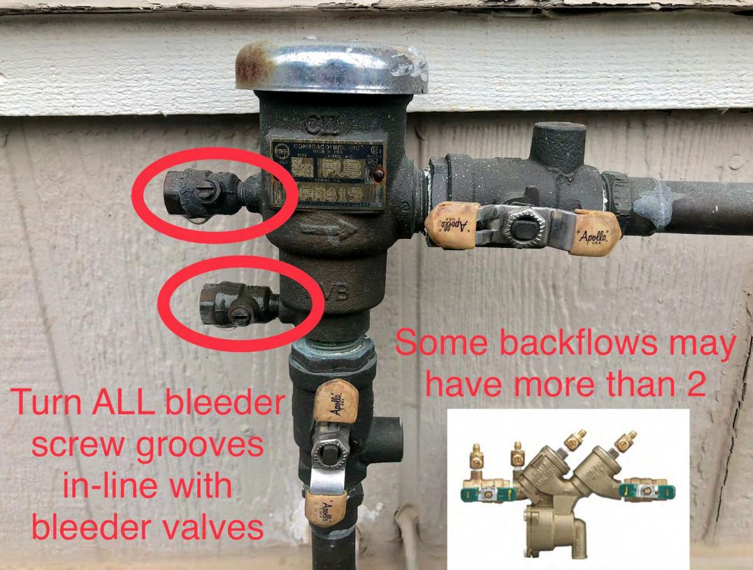
Return to your backflow and open **ALL bleeder valves** by turning the groove in the bleeder screw inline with the valve. Some may have more than 2, you need to open ALL valves. If you don't see the bleeder screw it may be on the backside of valve.
