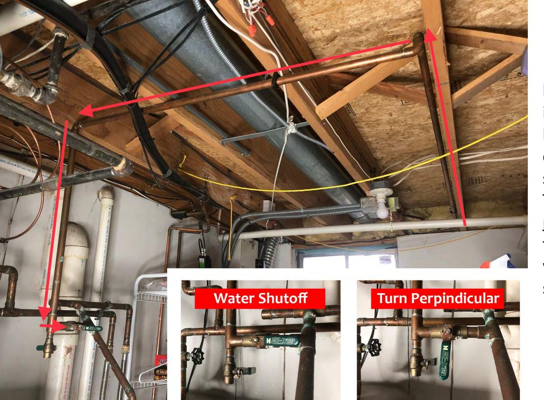
Follow the backflow pipe inside of your home until you come to the water shutoff handle. Turn the handle perpendicular to the pipe to shut the water off to your sprinklers.
