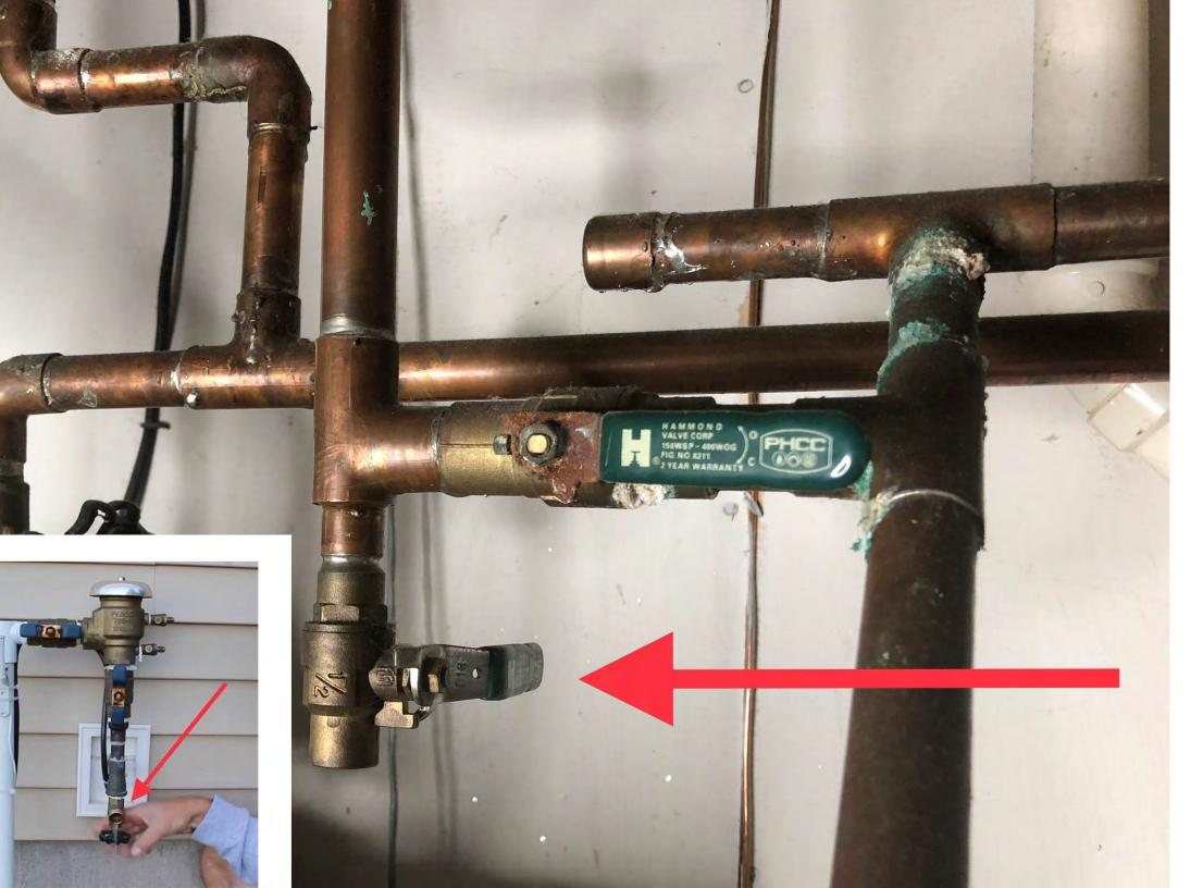
Locate the drain for your backflow. Some will be inside on the same pipe as the water shutoff and some will be outside on back flow itself. It will either be a handle or a wheel and will have an open end that's not connected to other pipes.
