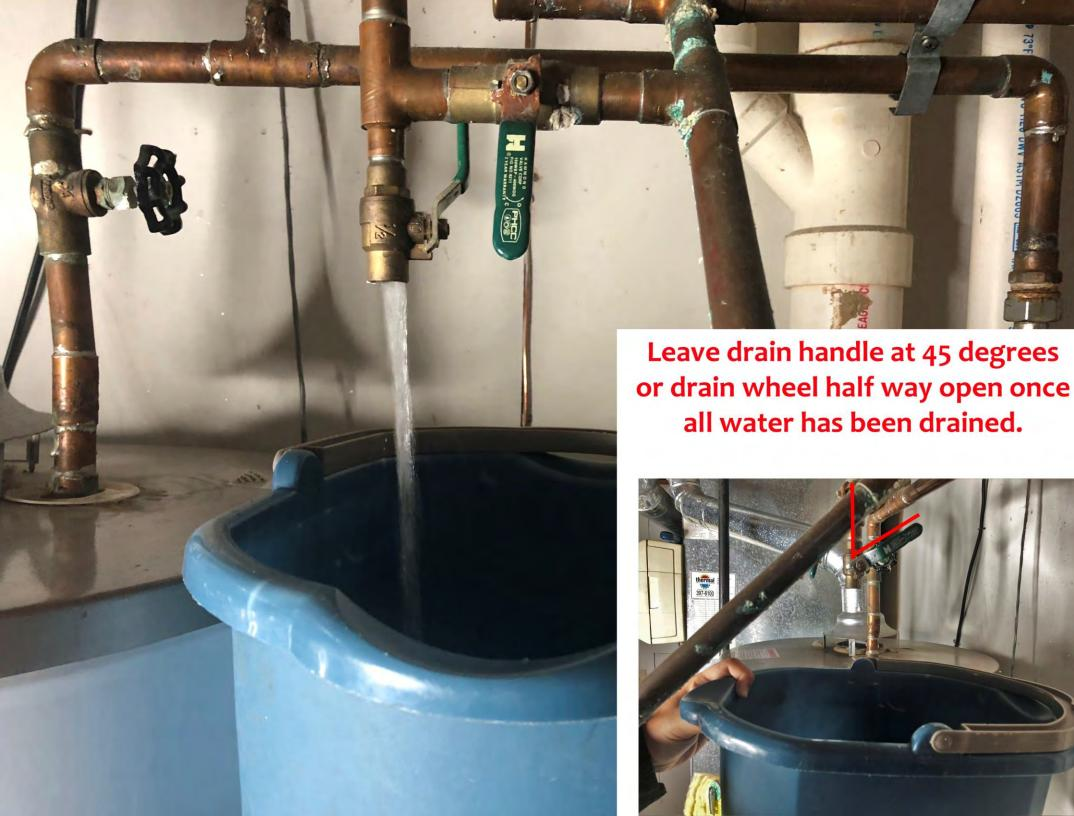
Place a bucket below your drain and open drain by turning handle inline with drain or by turning wheel all the way to the left. Once all water has been drained leave drain half open by turning handle to 45 degree position or by turning wheel halfway between open and close.
